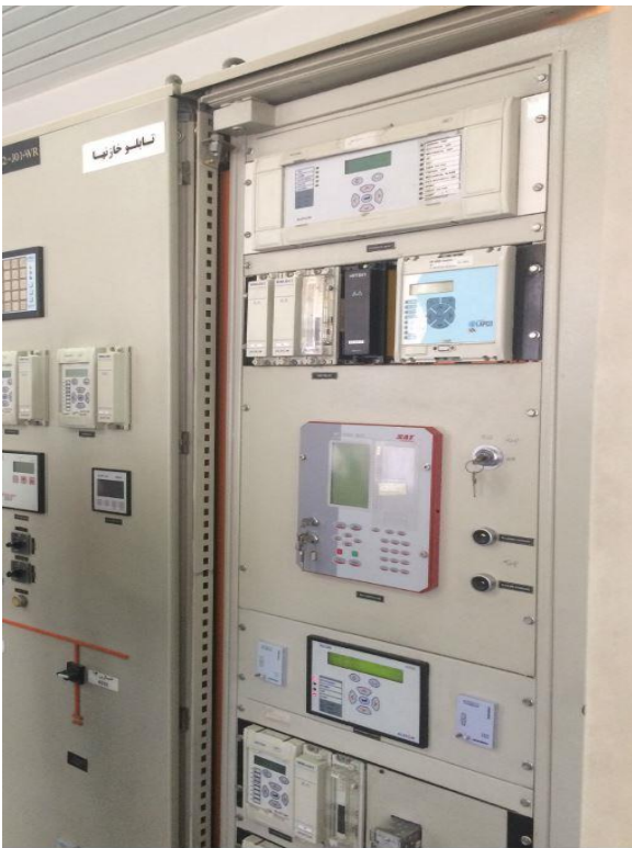
Pilot Installation of HF6028 relay on Balal Substation
