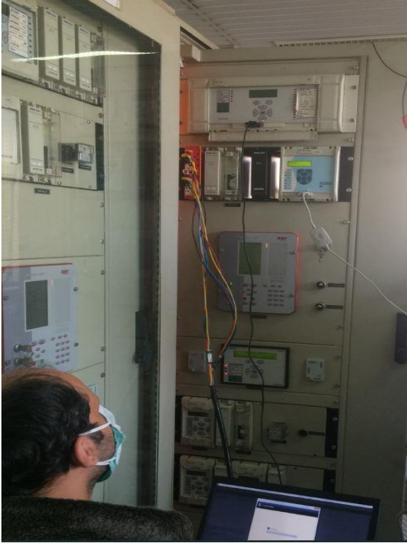
Pilot Installation of HF6028 relay on Sardar Jangal Substation
