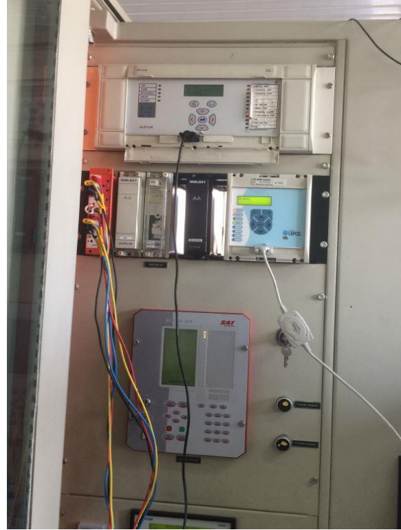
Pilot Installation of HF6028 relay on Sardar Jangal Substation
